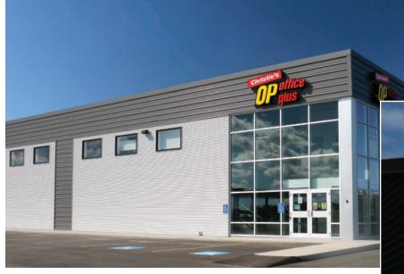
Easily installed over solid sheathing or open framing, 7/8" Corrugated can be lapped in a variety of ways, eliminating extra cutting on-site.
