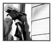
Exterior grade smooth shank nails can be used either nailed or shot. Exterior grade screws (#6, 8, and 10) are also acceptable. Any fastener used must be long enough to penetrate solid wood by no less than 1 1/4".
